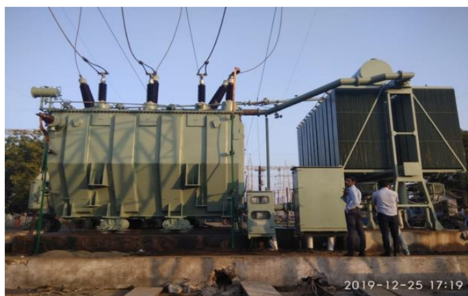
Figure:11 Transformer put back into service
