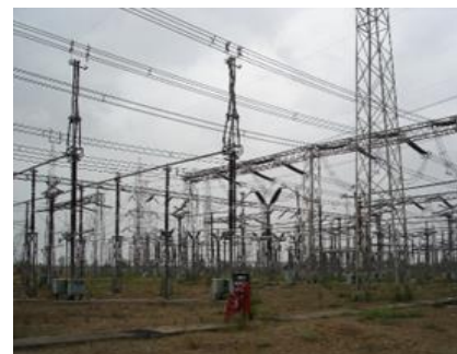
Image – 16 Portable Fire Extinguisher in Open
